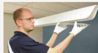
1. Lift and shift or remove the lens.
