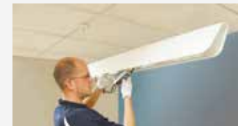
6. Remove the LED driver and replace.
