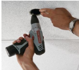
Using screwdriver (electric or manual), rotate installation screws in aperture to actuate pivoting installation arms. Arms will secure fixture directly to ceiling.
