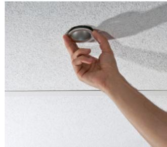
Align bumps on reflector housing with grooves in fixture body. Press flush to ceiling and rotate. Slight force is required to overcome initial resistance, ensuring proper installation.
