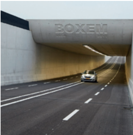
Tunnel entrance lighting
