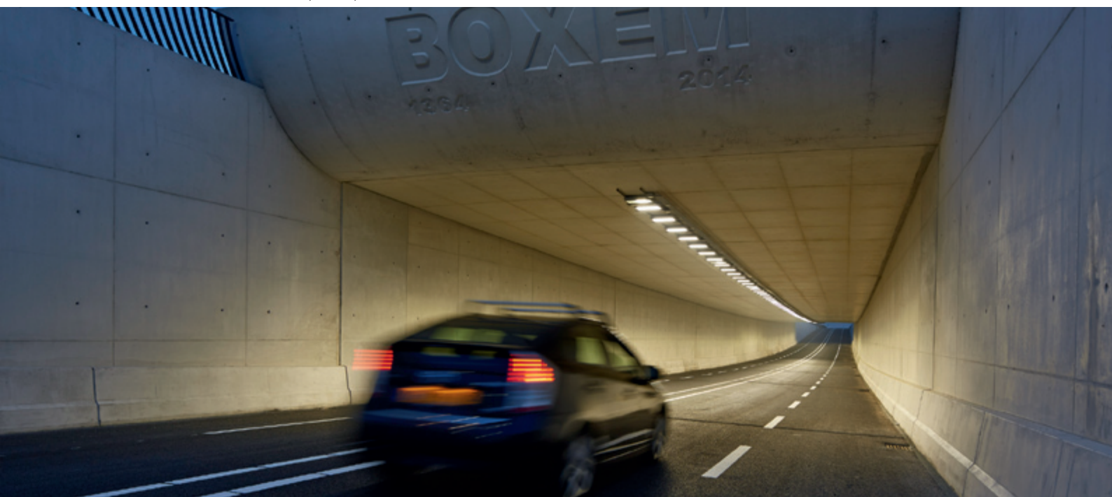
Boxumtunnel, Zwolle, The Netherlands
