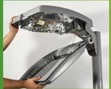
Unlatch and remove the existing door.
