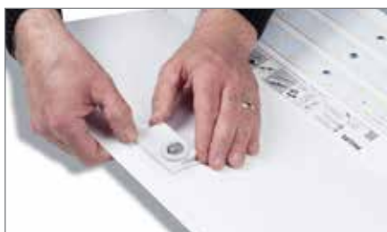
Step 5: Insert the sensor back into the hole. The sensor may or may not require a socket.
